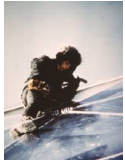
Putting in the rest of the node fasteners (NSF photo courtesy Jerry Marty)
