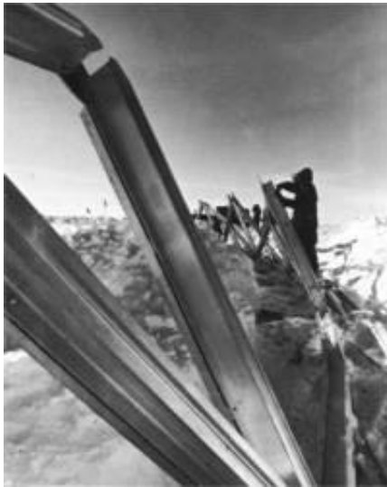
Seabees assemble the lower portions of the dome.
