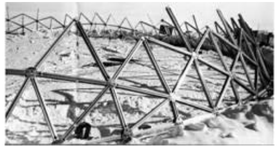
Seabees assemble the lower portions of the dome.
