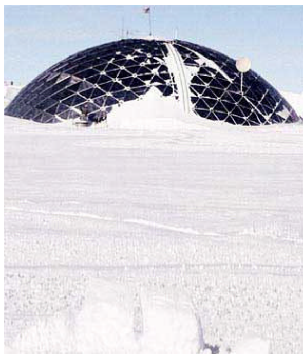
Photo by Amundsen-Scott South Pole Station Crew Today's central station, rebuilt in 1975; the main quarters are crowded underneath and aluminum done only 50 meters wide.
