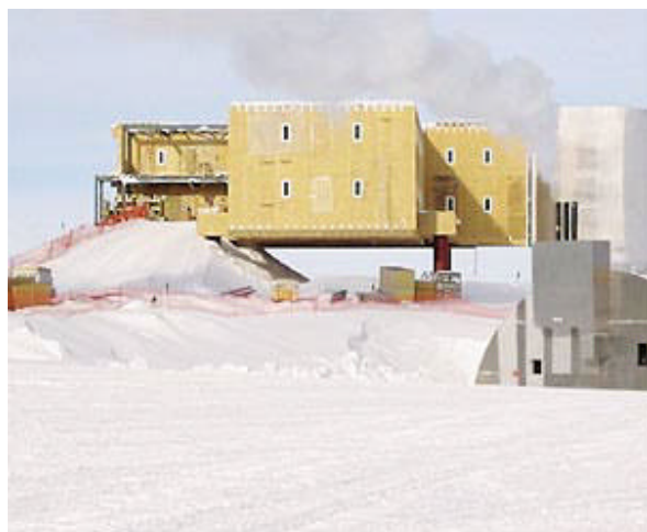
Photo by Amundsen-Scott South Pole Station Crew The elevated surface station will connect to the underground service area by a fully enclosed vertical tower.
