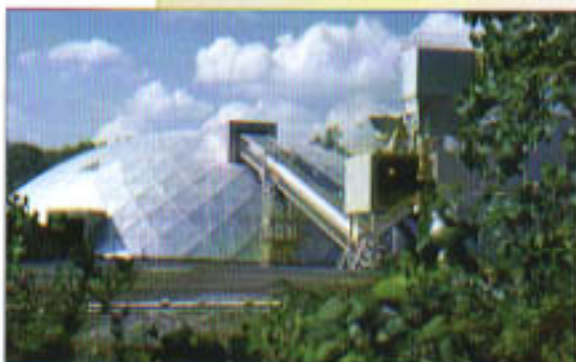
Temcor's dome at St Lawrence Cement
