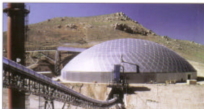
A 102m Temcor dome on a 6.1m steel wall frame Monolith, CA, similar to the dome being built at the AES Total Energy Plant
