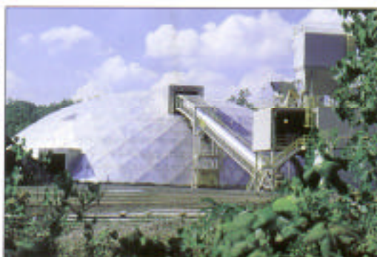
Hagerstown cement storage dome
